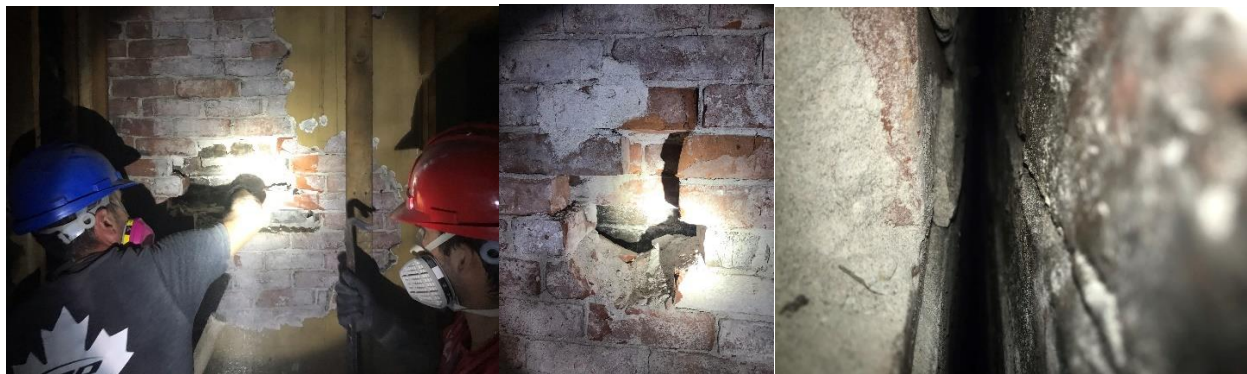
Figure 5 – Investigation of the wall interface
