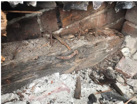
Figure 7 – Rafter nailed to neighbouring building
