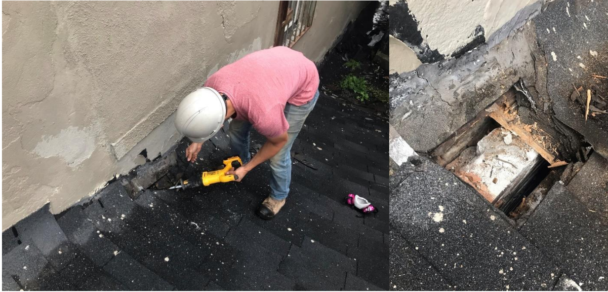
Figure 6 – Investigating the roof interface
