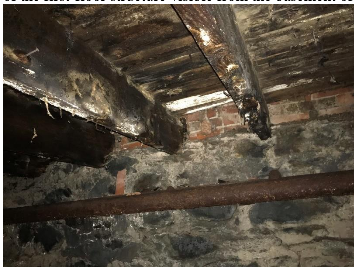
Figure 14 – Structural decay in the basement
